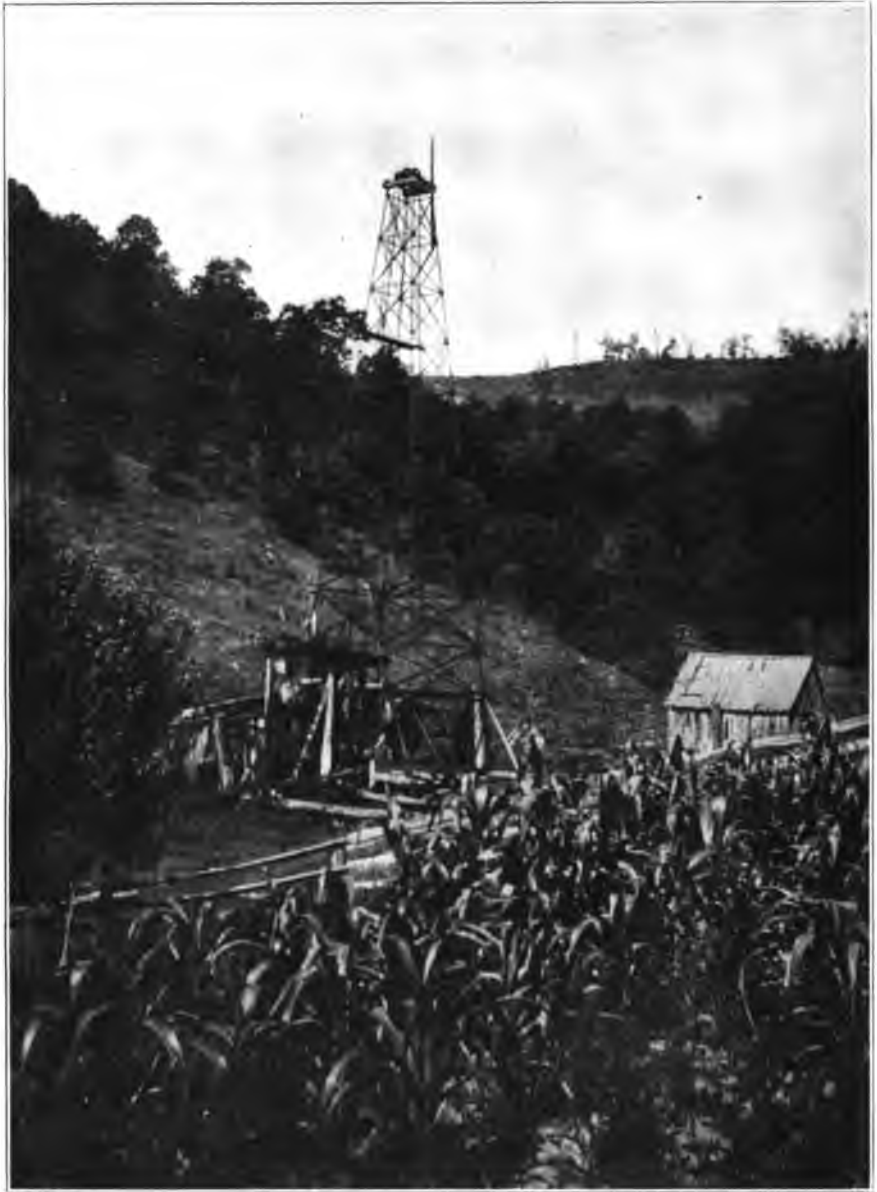
PLATE XVII.—Steel-tube Derrick used by the South Penn Oil Co.— McIntyre well (356), 2½ miles south from Rinehart —and Dunkard series Topography.
